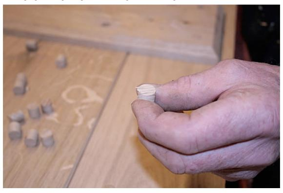
Hammer the oak plug into the plug hole, leaving about 5mm of the plug proud of the ledge surface.
