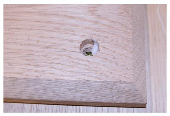
Take an oak plug and align its grain with the grain in the ledge.
