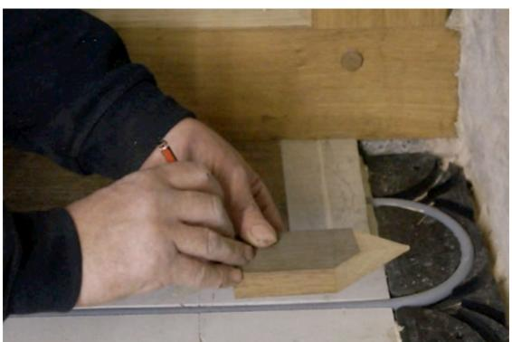
With the pointed edge against the wall and the pencil held in place by the groove, slowly run along the wall drawing the outline onto the masking tape covering the end of the floorboard. This will give an identical representation of the wall's undulations, marking where you will need to cut.
