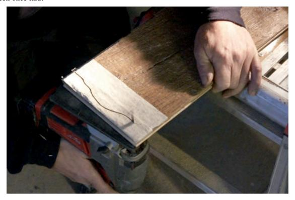
Now that the scribe has been marked and cut, the final job is to check that the scribe has worked. To do this, simply slide the board into place so that it fits perfectly up against the wall.
