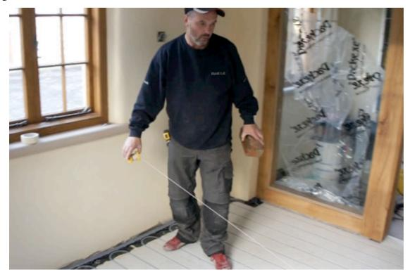
We can do this by creating what is known as a **datum line** which stretches across the room and works as a reference point to check that the walls are parallel.
