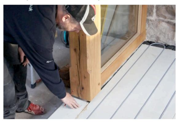
To check that there are no problems later on, measure from the marked line to the other side of the room. Check to ensure that you are not going to be left with a very small width of board at the end.
