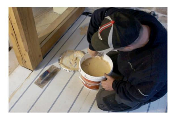
Before trowelling the glue on, it is important to check the consistency of the glue to ensure it creates a nice smooth finish. Any hard "crusted" areas should be removed beforehand so that they do not affect the adhesion.
