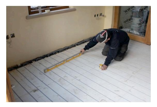
Once it has been established that the sub-floor is dry enough, the next job is to check that it is reasonably level. This should be done using a spirit level, which should be placed at various intervals around the room. The levels should not vary more than +/- 2mm per metre. Check the edges of the room for rises and dips, ensuring you have a flat, even surface to work from.
