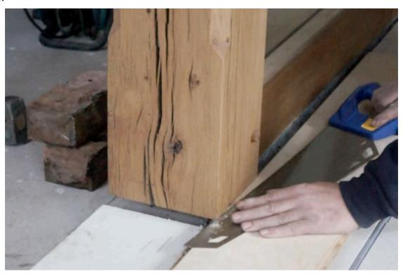
We did this by taking an off-cut of one of the oak boards and turning it upside down. The board was placed next to the frame, which we marked using a handsaw. We repeated this process for all sides of the frame. Once marked, the partition frame was cut using an electric saw.
