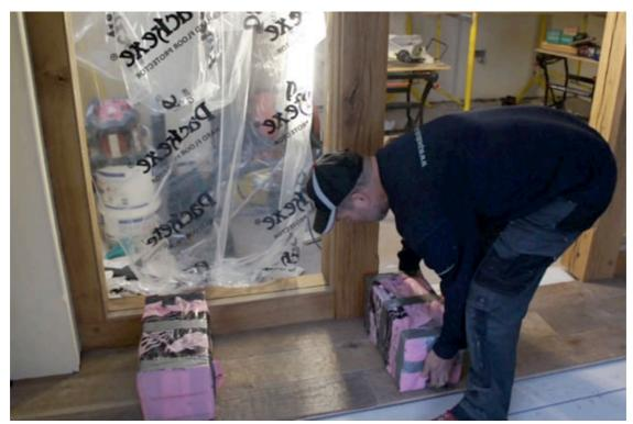
Simply repeat the process of trial fitting a few rows of floorboards, marking the sub-floor, lifting the boards, applying the glue, re-laying the boards and weighing them down until the whole room is complete.
