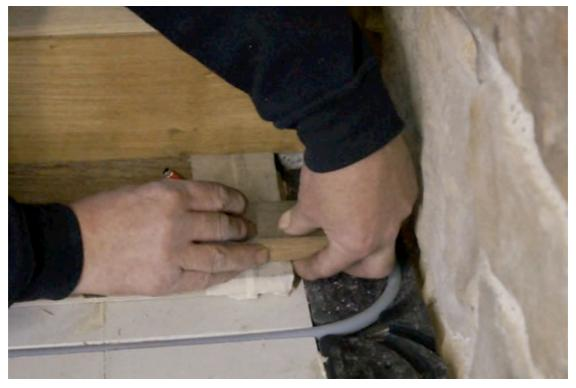
Begin by placing a small amount of masking tape over the edge of the board to be scribed.
