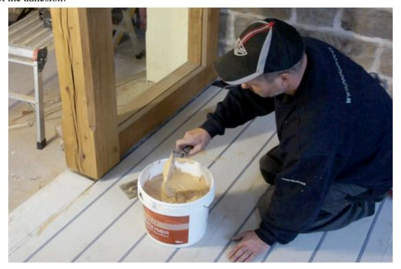
You can now begin to trowel your glue onto the sub-floor. In this example we have used a 6mm grooved trowel to apply the adhesive. When the trowel is standing upright the grooves are 6mm, however when trowelling you will normally work at a 45 degree angle, which in reality makes the height of the notch only 3mm. We believe this height gives much better adhesion between the board and sub-floor.
