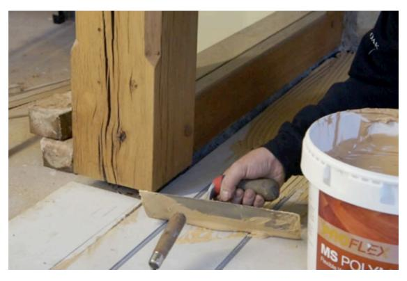
Please Note: When applying the adhesive make sure to not go over the marked lines, but instead slightly back from them to avoid problems if the glue sets before the next set of boards are laid.
