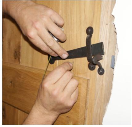
Drill a hole through each of the marks and then join the holes to create one large hole, big enough for the latch bar to fit through.
