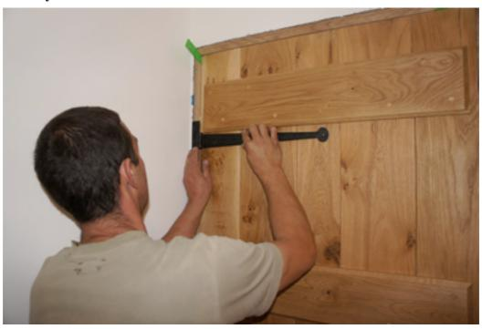
Once aligned, drill pilot holes through the hinge into the door casing/frame.
