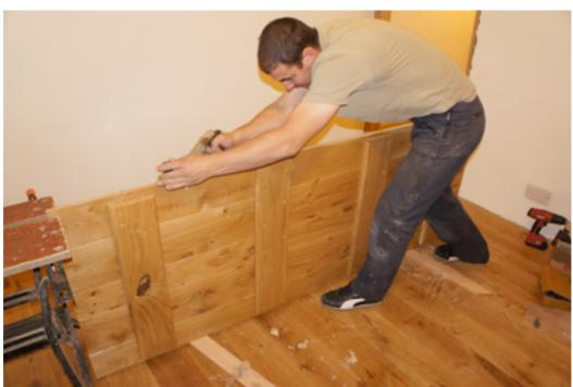
Using a hand plane, remove the marked areas a little at a time and keep trial fitting until the gaps are even around the entire door.
