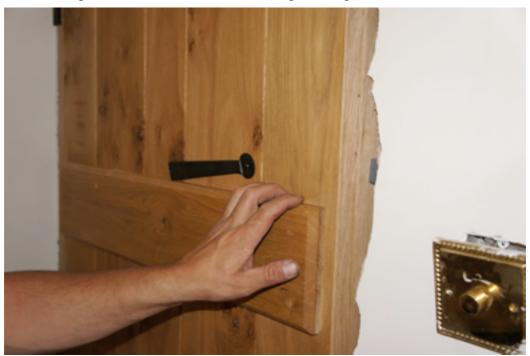
Next, line up exactly where you would like the clasp to be placed on your door frame in relation to the bar.
