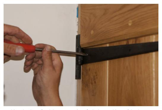
Once the top hinge has been fitted the next step is to fit the bottom hinge of the door.
